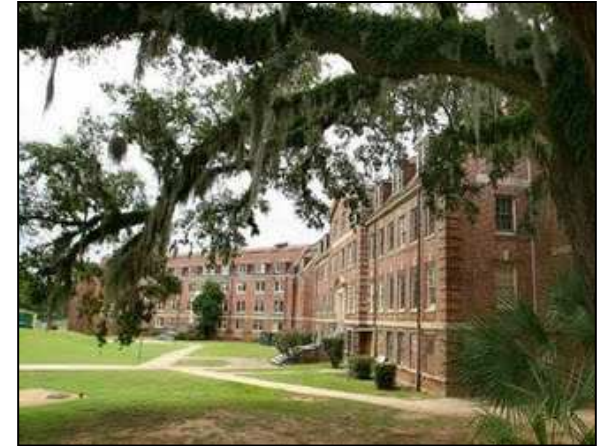
Florida A&M University Sampson Hall and Young Hall Dormitories Tallahassee, Florida
