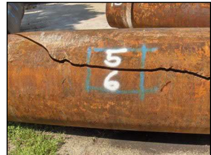
FKAA Transmission Main Replacement Key West, Florida
