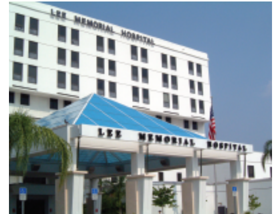
Lee Memorial Hospital ER Expansion Fort Myers, FL
