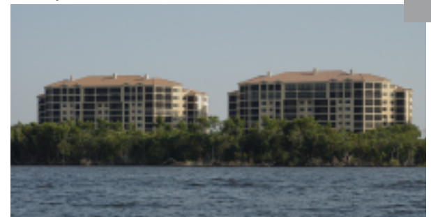
Palmas del Sol High Rise Condominiums Fort Myers, FL
